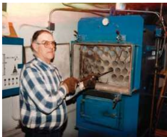
Manual boiler tube cleaning at Calais Elementary School, Calais, Vermont (from the Biomass Energy Resource Center's Wood Chip Heating Systems)
